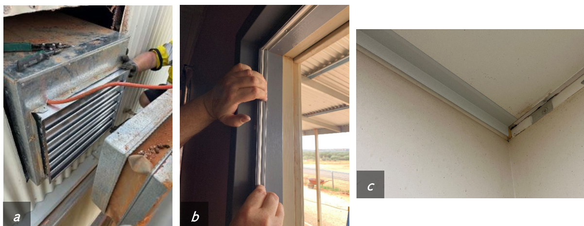
Figure 15. Example upgrades to address airtightness issues: (a) damper installed in evaporative cooling system; (b) door seal; (c) new cornice detail, applied to linings with caulking.
