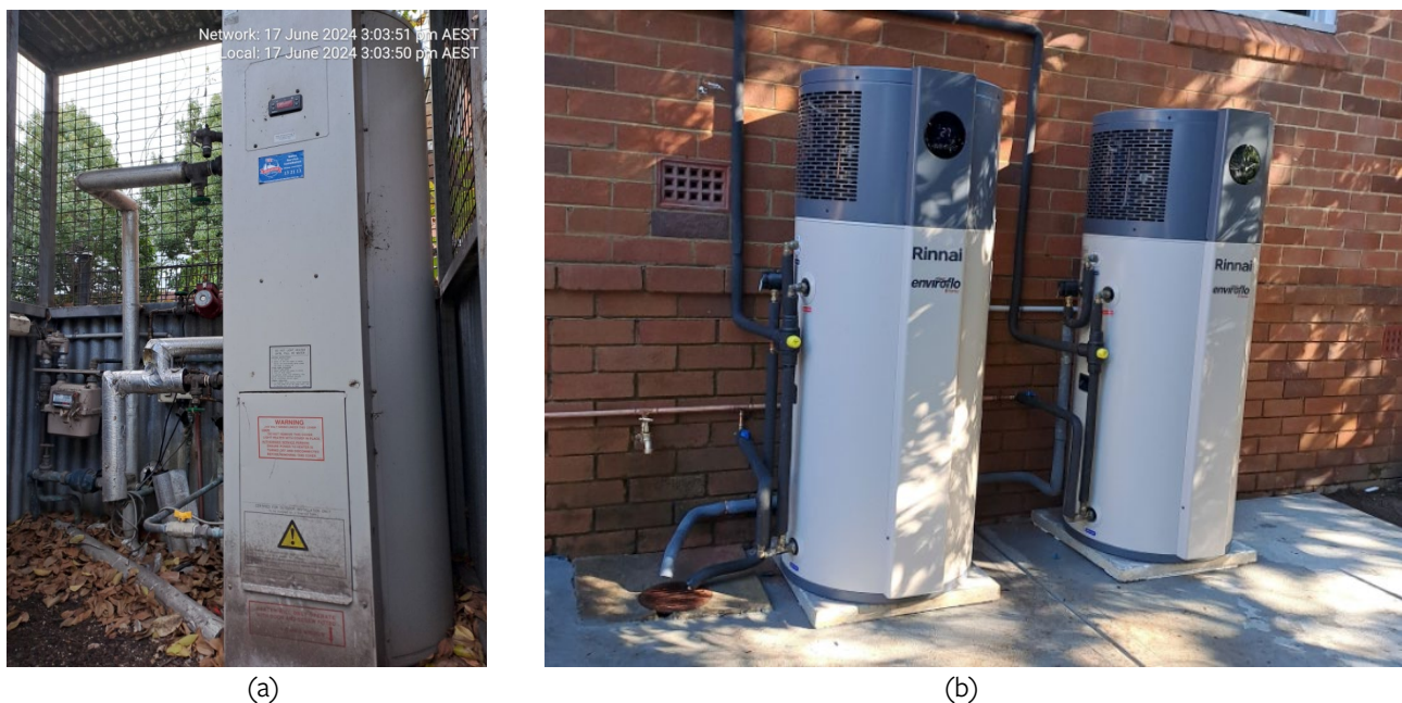
Figure 23. (a) Common gas-fired hot water systems were replaced with (b) individual heat pumps for two unit complexes in Sydney as part of an electrification upgrade.
