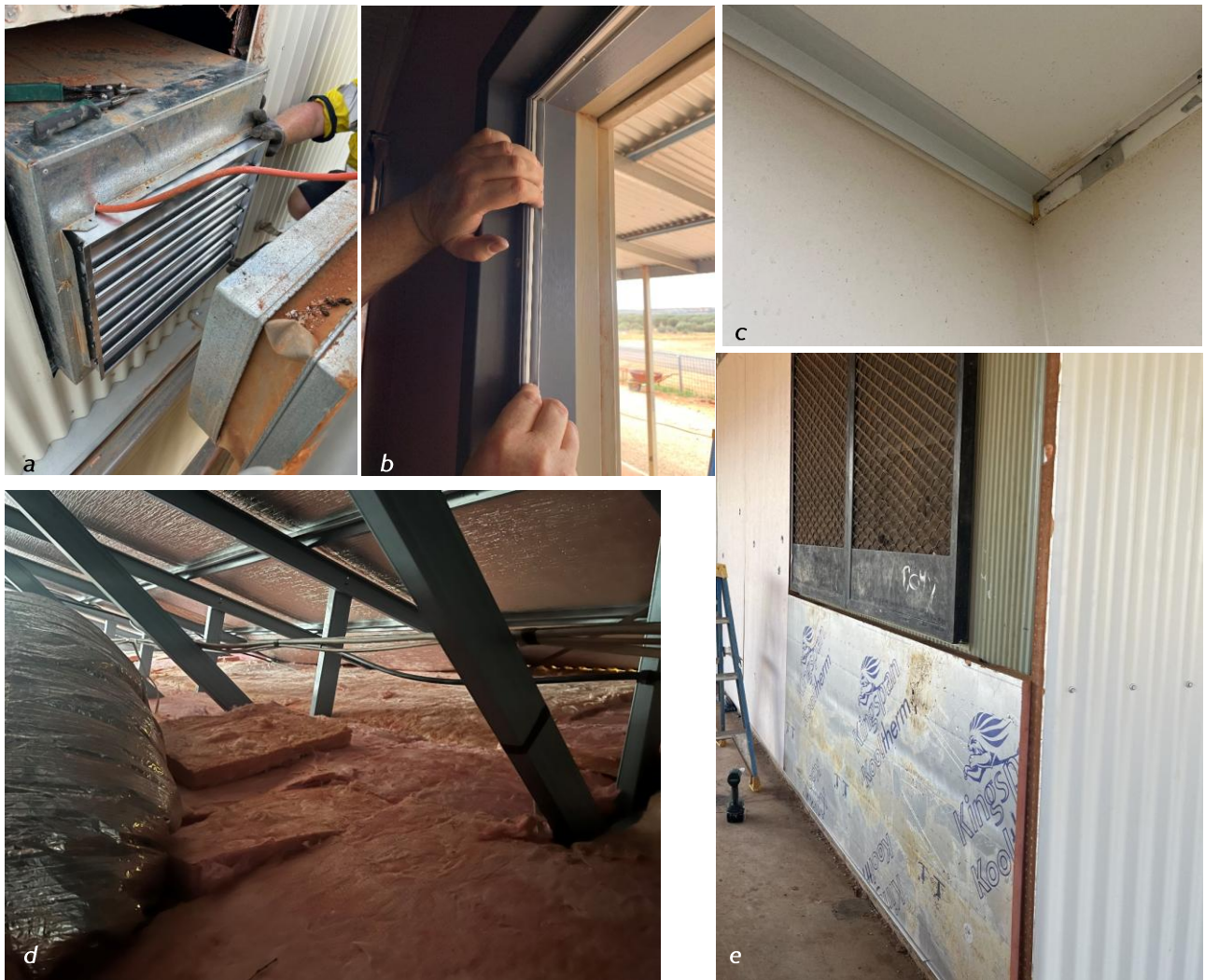
Figure 8. Examples of airtightness upgrades and thermal bridging mitigation measures: (a) damper installed in evaporative cooling system; (b) door seal; (c) new cornice detail, applied to linings with caulking; (d) semi-rigid glasswool covering roof truss bottom chords; (e) rigid foam board added to external walls.
