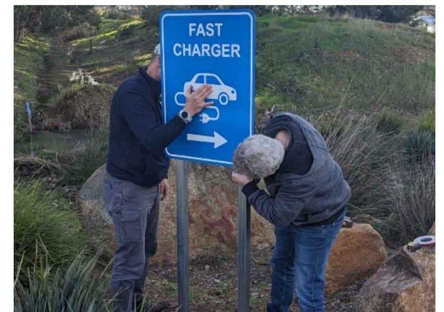
Figure 11: Installation of signage at the entrance of the village as part of the research intervention
